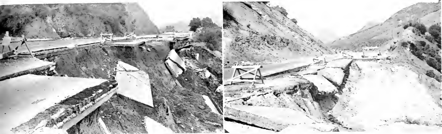
Views of slipout on Ridge Route Alternate, U. S. 99. Sketch shows method of correction
